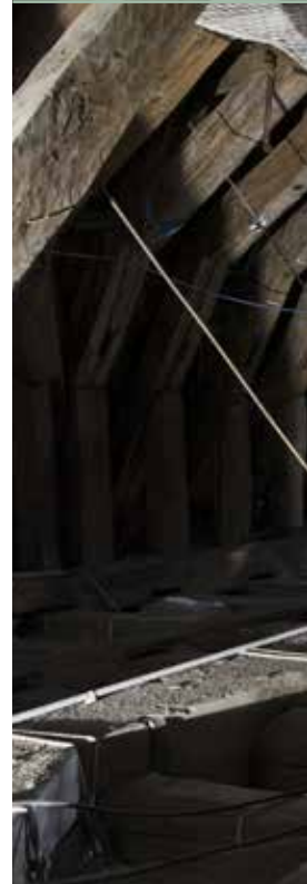
Current state of the roof beams of the Royal Chapel, 2016.
